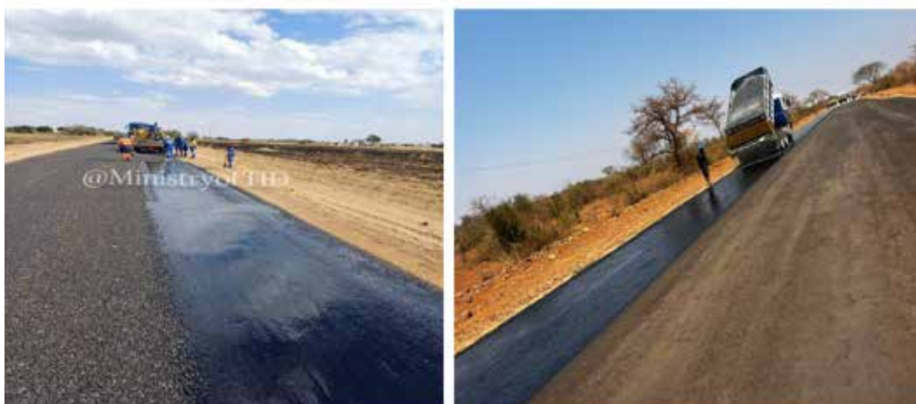
Resealing of Chivhu – Gutu Road and surfacing of Bulawayo – Nkayi road
