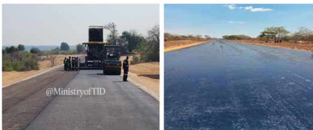
Surfacing of Murambinda – Birchenough Road and Priming of Murewa – Madecheche road
