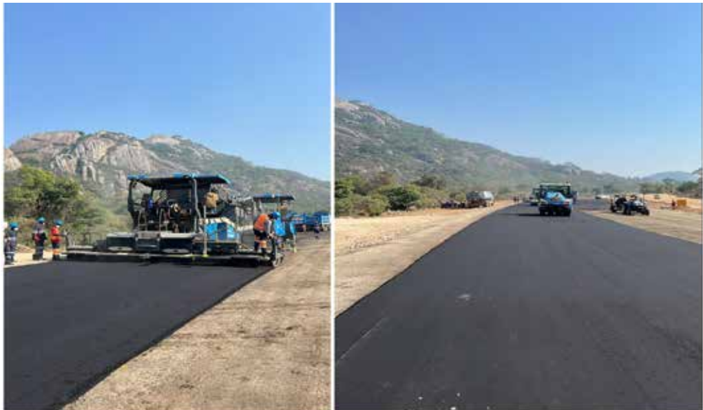
Surfacing on the Harare-Masvingo-Beitbridge Road (Ngundu Section)
